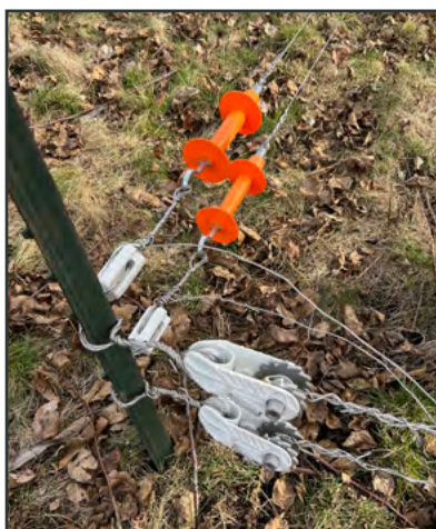
A corner T-post with strain insulators, tighteners, and gate handles. A hot wire bridges the corner to carry the electricity past the post and insulators.
