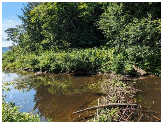
Beaver Deceiver™ Device installed at a beaver dam in Charlotte
